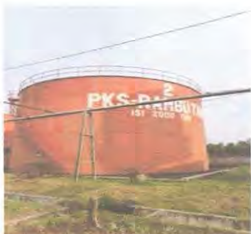
Gambar 3. 29 Oil Storage Tank
