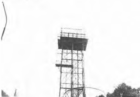
Gambar 3.38 Water Tower Tank
