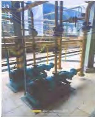
**Gambar 14. Oil Pump final Transfer**
