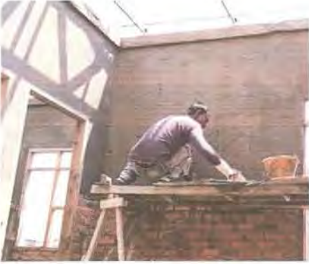
Gambar.2 Proses plasteran
