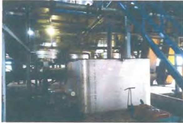
Gambar 3. 19 Crude Oil Tank
