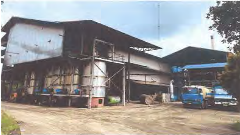
Gambar 2.1. Pabrik Kelapa Sawit PT. Mulia Tani Jaya
