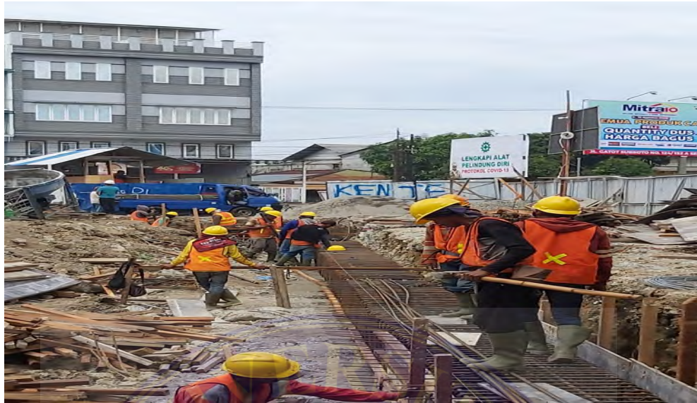
Gambar 3 Proses Pembesian Dinding Penahan Tanah
