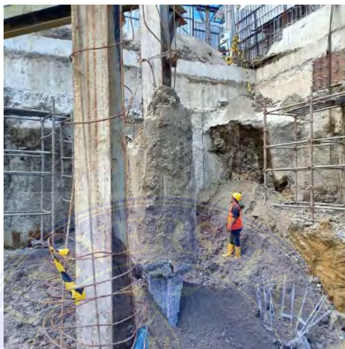
Gambar 1. Bore Pile
