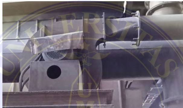
Gambar 2.3 Carrier Air Fan (Sumber: PT Socfindo)
