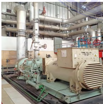
Gambar 2.5 Turbin Uap di PT Socfindo) (Sumber: PT Socfindo)
