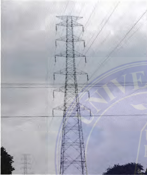
Gambar 2.4.a Tower 4 sirkit tipe suspensi (Suspension Tower)
