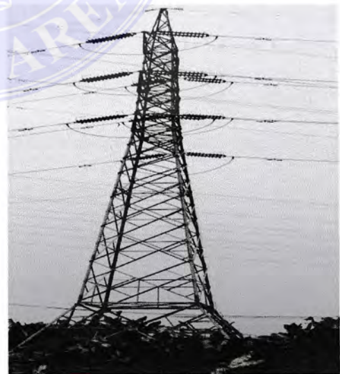
Gambar 2.5.b. Tower 2 sirkit tipe tension
