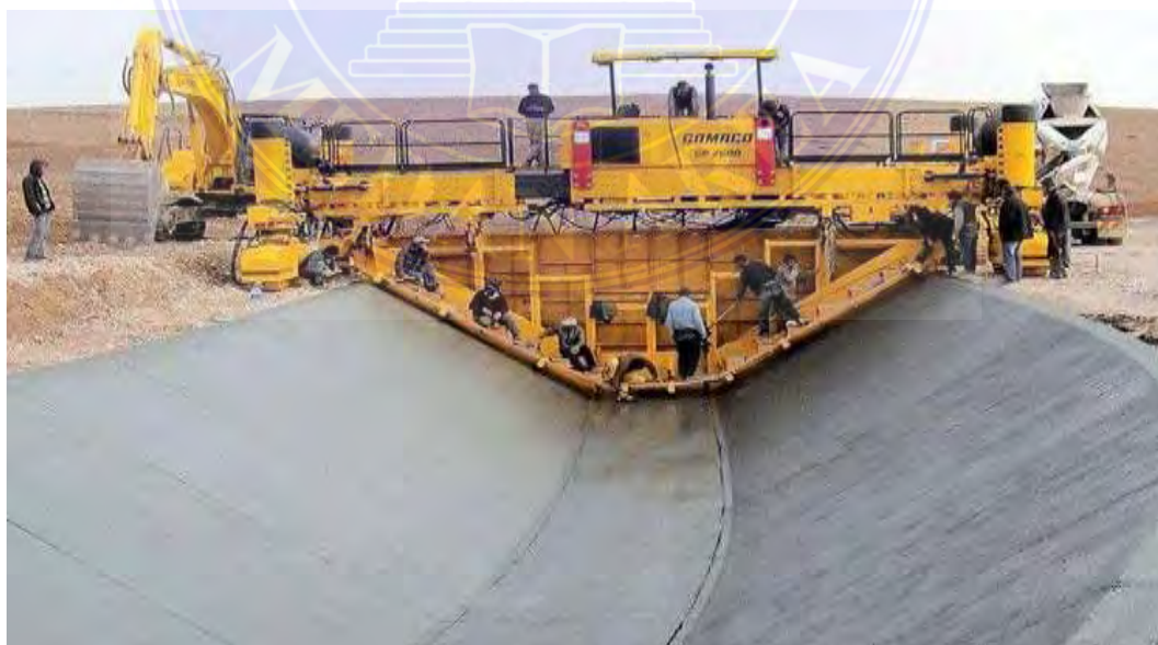
Gambar 12. Transverse Concrete Finishe (Ady Sanam ,2012)
