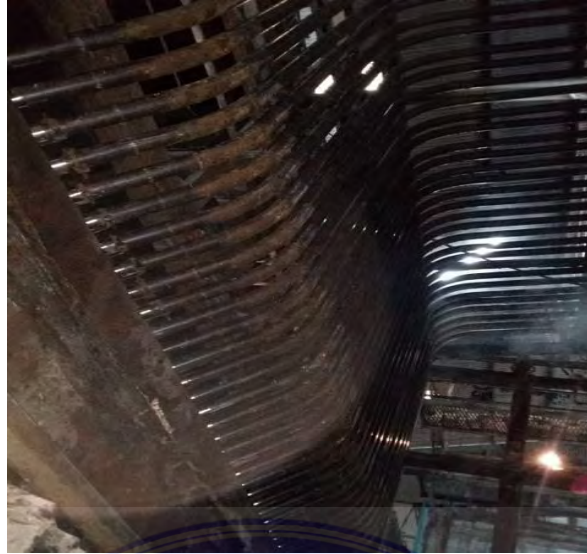
Gambar 2. 7 Pipa Superheater
