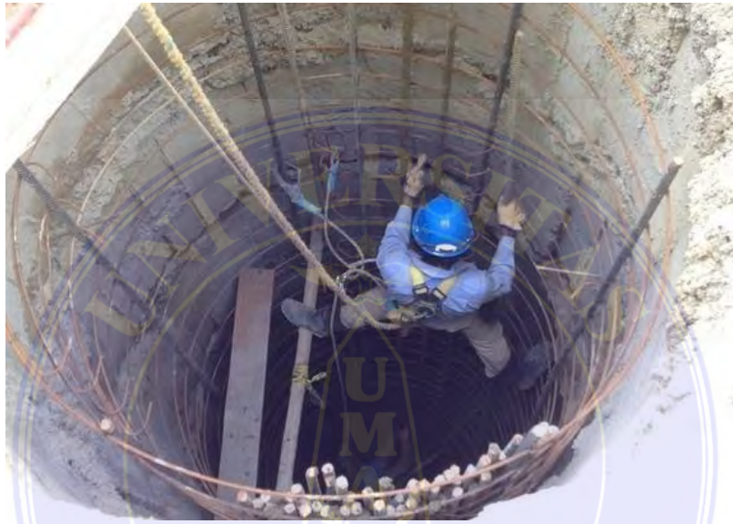
Gambar 4.1 Pondasi Sumuran ( pier foundation ) (Hardiyatmo, 2002)
