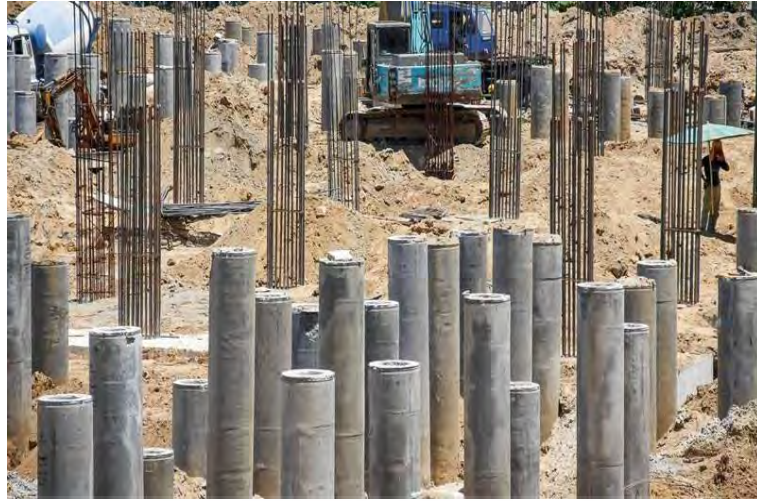
Gambar 5.1 Pondasi tiang ( pile foundation )( Mohammad Yani,2022 )
