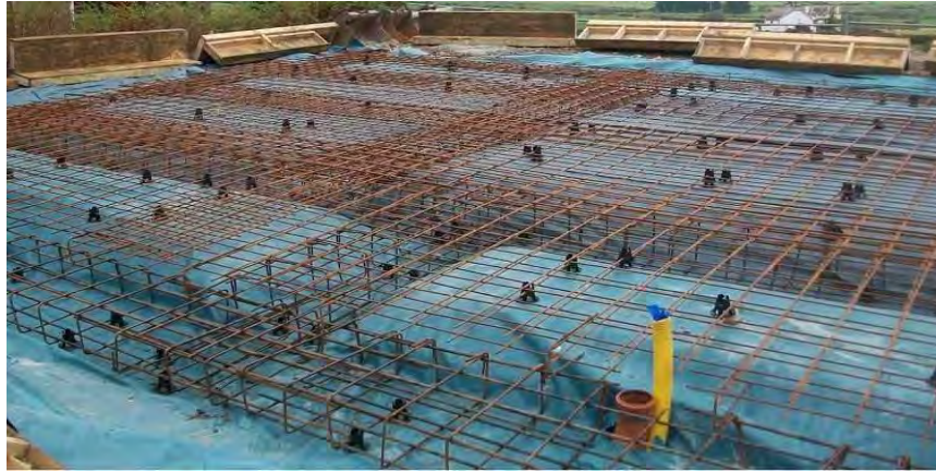
Gambar 3.1 Pondasi Plat ( raft footing ) (Chairrunissa, 2018)
