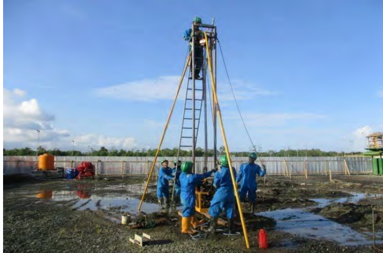
Gambar 8.1 Bore pile Gawangan ( Chairunissa )
