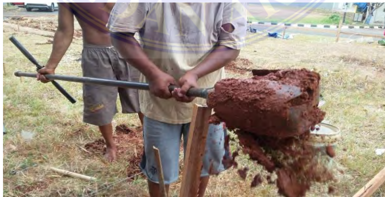
Gambar 9.1 Bored pile Manual/ Strauss .( Lapangan Sipil)
