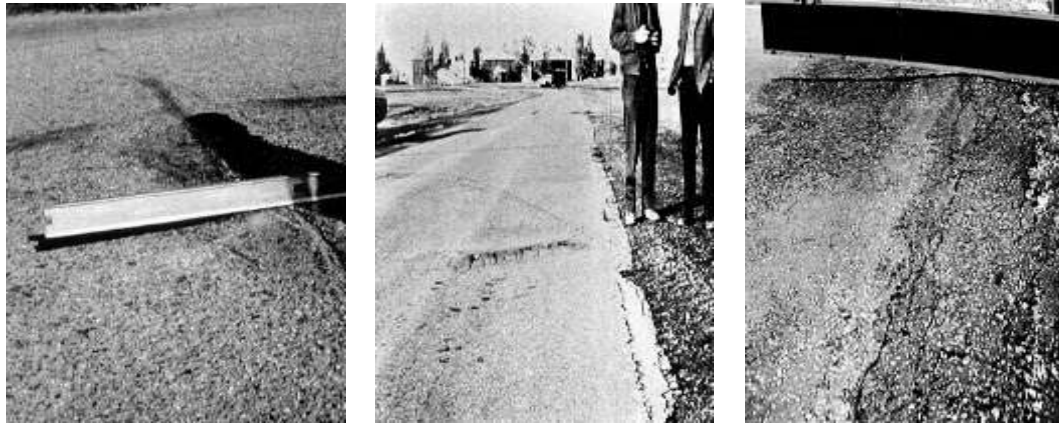
(a) Low (L) (b) Medium (M) (c) High (H) Gambar 6. Cekungan ( bump and sag ) (ASTM International, 2017)
