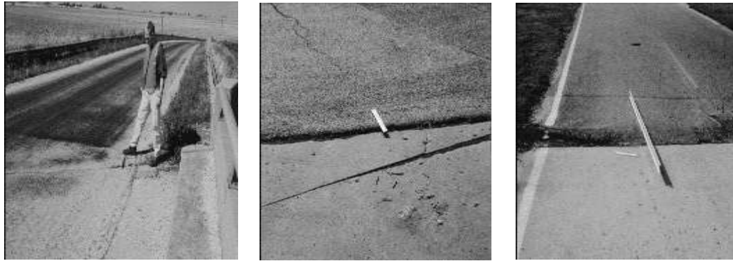
(a) Low (L) (b) Medium (M) (c) High (H) Gambar 18. Sungkur ( shoving ) (ASTM International, 2017)
