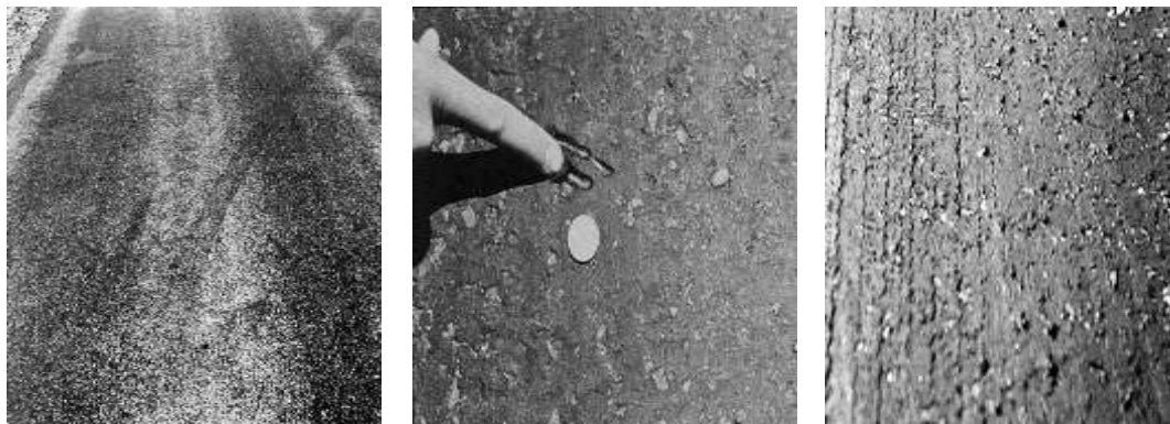
(a) Low (L) (b) Medium (M) (c) High (H) Gambar 4. Kegemukan ( bleeding ) (ASTM International, 2017)
