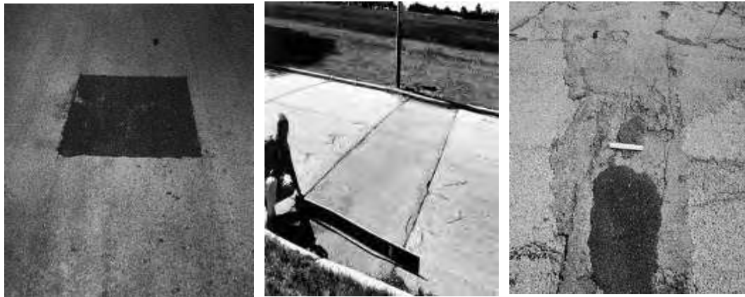
(a) Low (L) (b) Medium (M) (c) High (H) Gambar 13. Tambalan dan galian utilitas ( patching and utility cut patching ) (ASTM International, 2017)
