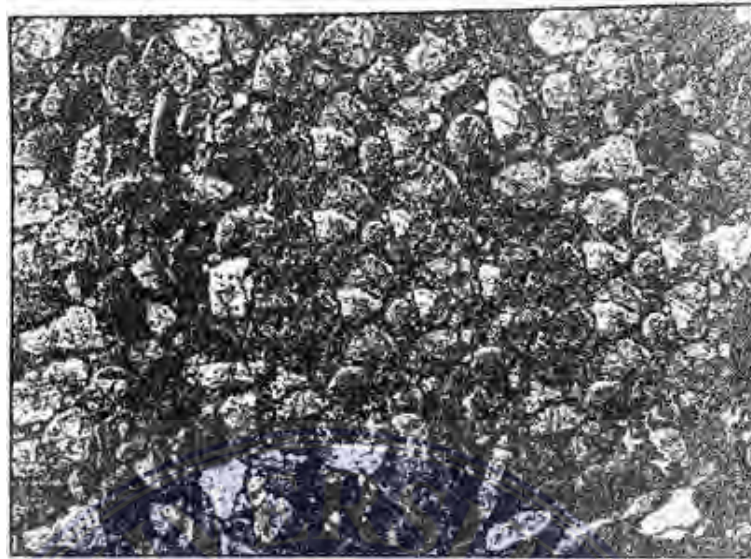
Gambar 39. Kerusakan agregat licin ( polished aggregate ) (Hardiyatmo, 2015)
