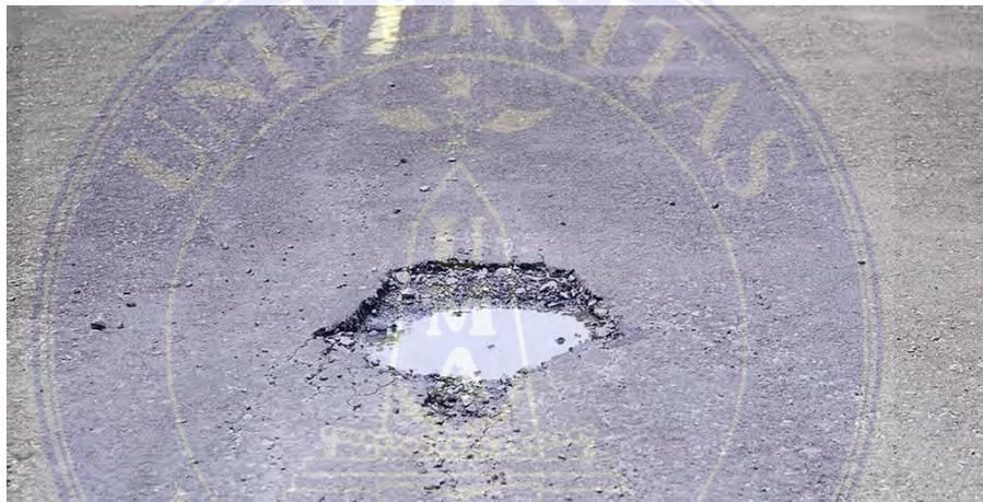
Gambar 11. Lubang *Pothole* ( Binar Maga No. 03/MN/B/1983)
