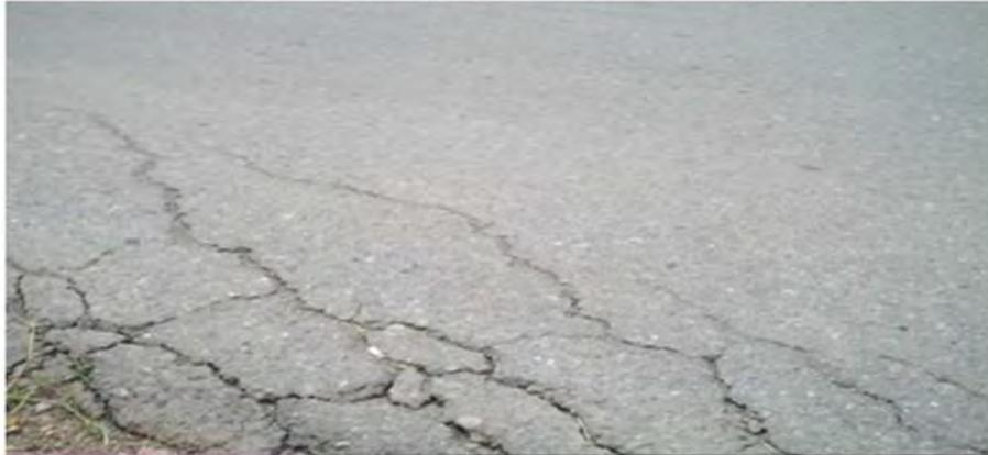
Gambar 2. Retak kulit buaya *Alligator Crack* (Binar Maga No. 03/MN/B/1983)
