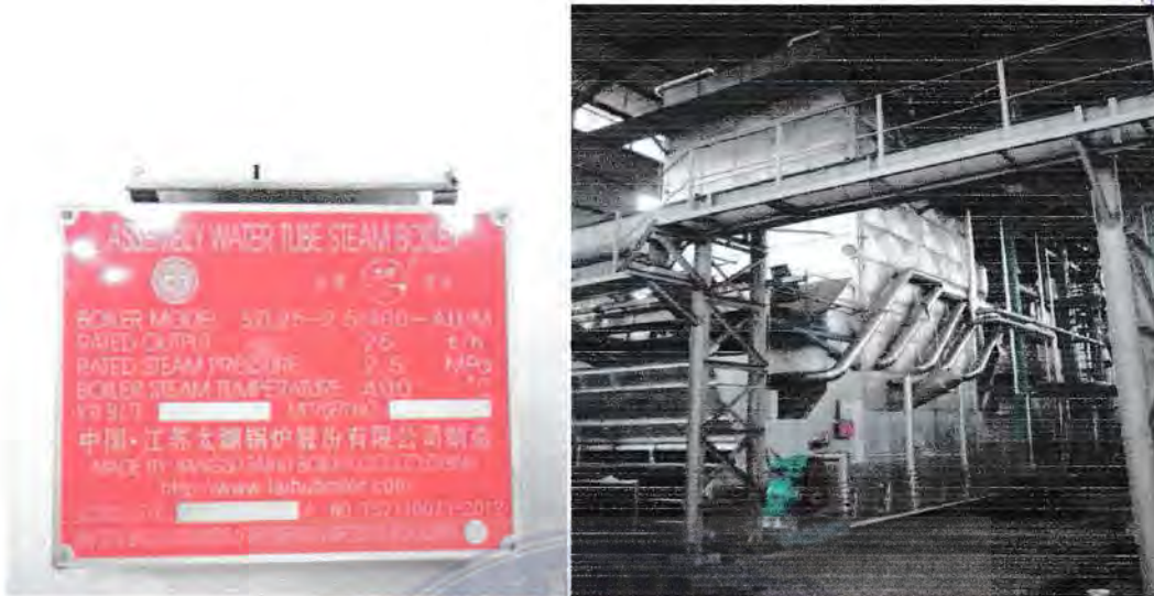
Gambar 2.3.2. Ketel Pipa Air ( PT. AJP )
