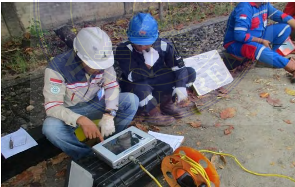
Gambar 10. Pelaksanaan pengujian PDA test ( pile drive analysis )
