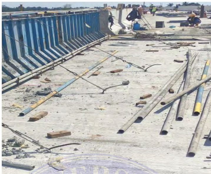
Gambar 1. Barrier/parapet (PT. PP, 2021)
