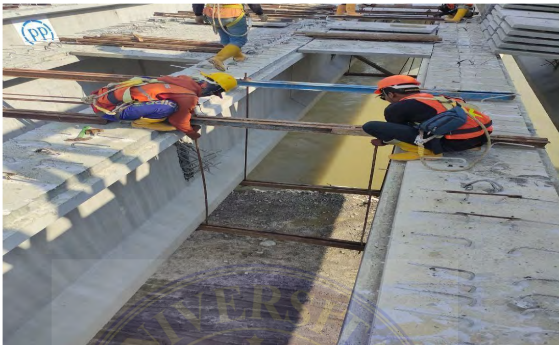
Gambar. Pengukuran Bekisting Diagrama (PT. PP, 2021)
