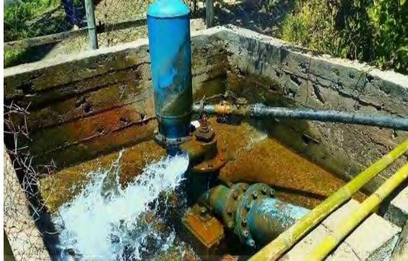
Gambar 2.3. Hydraulic Rump
