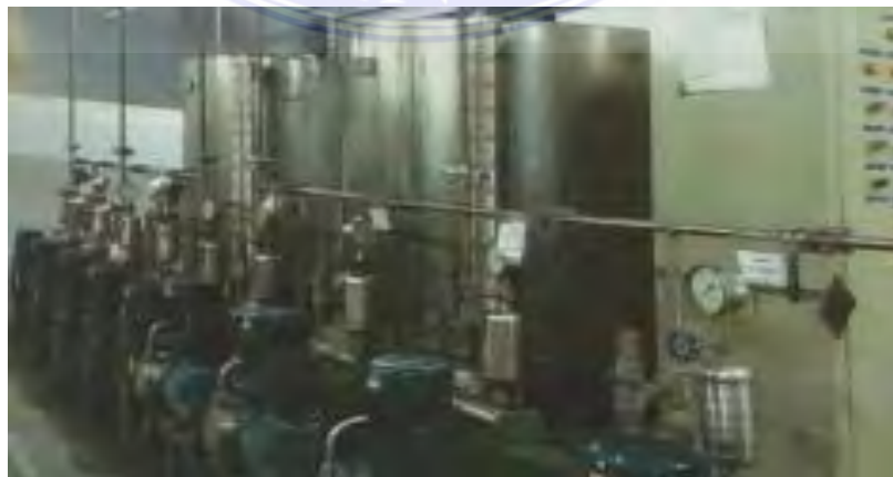
Gambar 2.14. Hydrazine Pump
