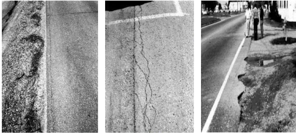
(a) Low (L) (b) Medium (M) (c) High (H) Gambar 5. Retak pinggir ( Edge Cracking ) (ASTM International, 2018)
