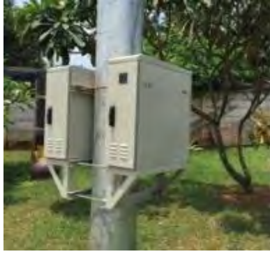
Gambar 2.8: Box control BTS outdoor
