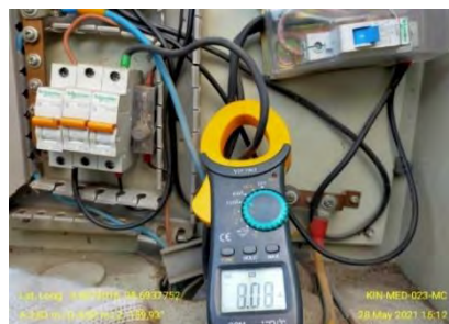
Gambar 3.8: Load (Beban) Phase R (Photo)( KWH - ACPDB)
