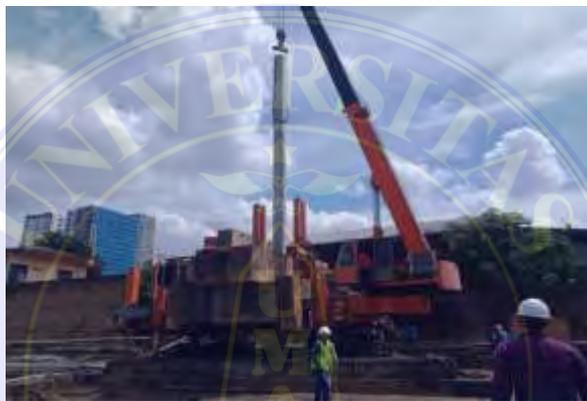
Gambar 3.10 *Hydraulic static pile driver*
