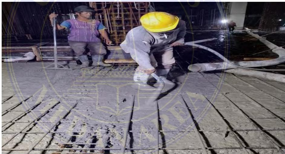
*Gambar 3. 12 Concreate Vibratrion*
