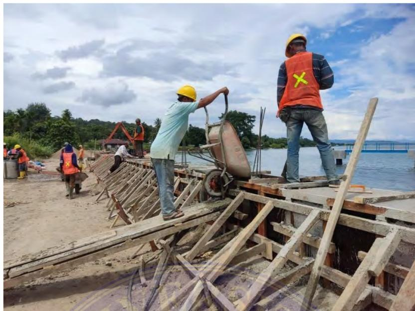
Gambar 4.13 Pengecoran *Capping beam*
