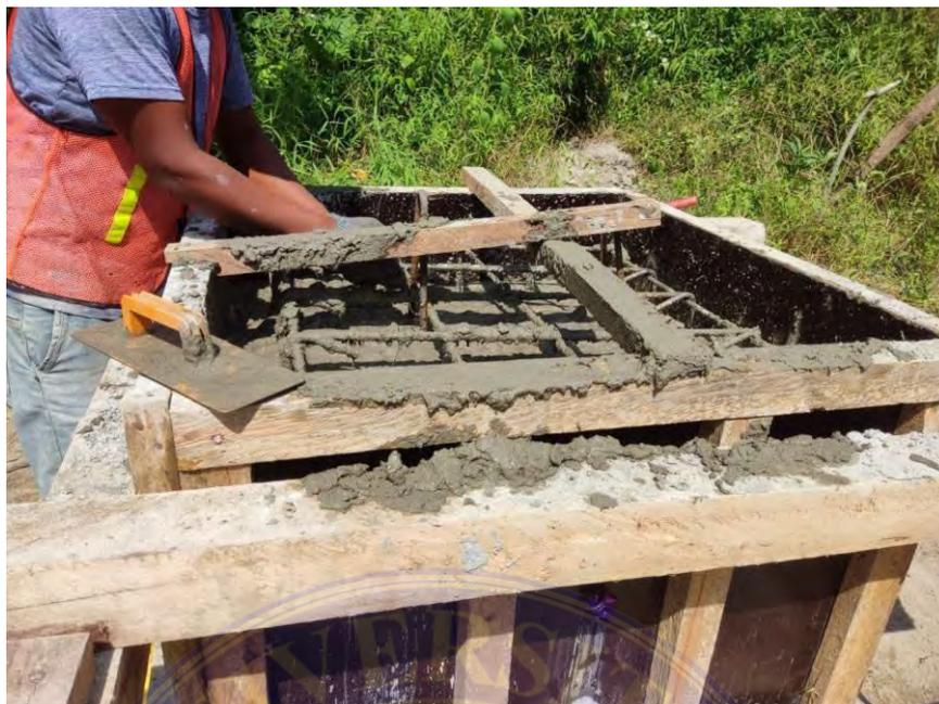
Gambar 4.15 Pengecoran *Counter Weight*
