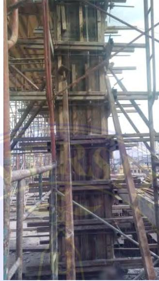
Gambar 4.4 Bekisting Kolom
