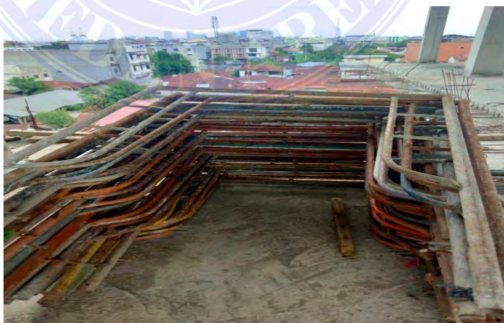
Gambar 3.19 Scaffolding Sumber : Data Lapangan
