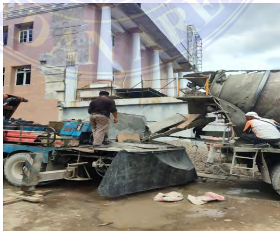
Gambar 3.9 Truck Mixer Beton Sumber : Data Lapangan
