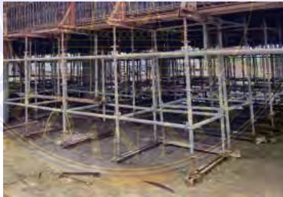
Gambar 3. 24 PCH System Ring Lock Sumber : Data Lapangan
