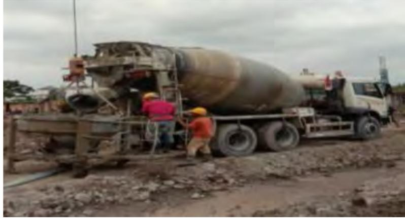
**Gambar 4.8 Menuangkan Beton Read Mix Ke Concrete Bucket 1**
