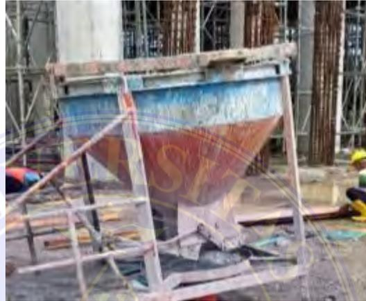
**Gambar 3.21 Concrete Bucket 1**
