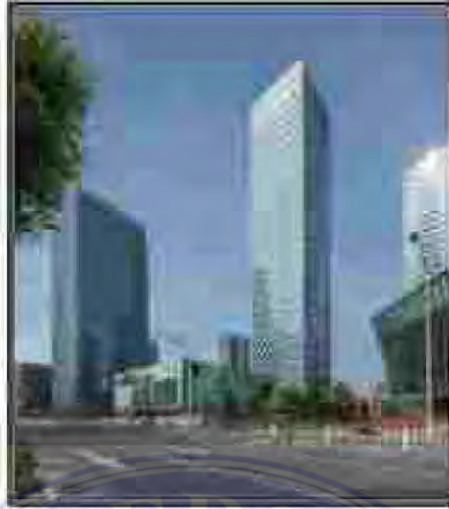
Gambar 2. 5 Beijing Green Land Center. (Sumber : ArchDaily.com)
