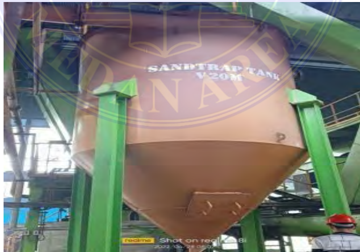
Gambar 3.5. Sand Trap Tank
