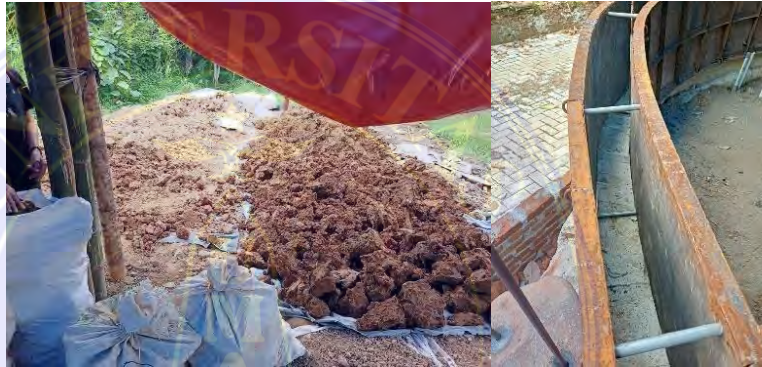
Gambar 3. 11 kiri tanah, kanan bekisting
