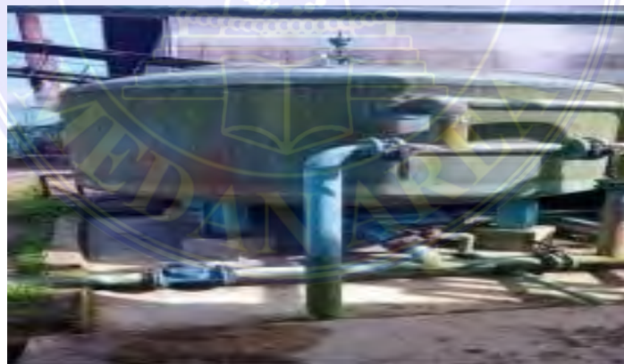
Gambar 3. 26. Sand Filter
