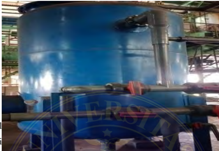
Gambar 3.29. Anion Exchange Tank
