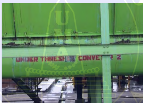
Gambar 3.25. Under Thresher Conveyor
