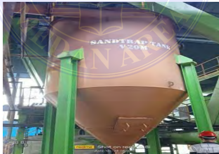
Gambar 3.5. Sand Trap Tank
