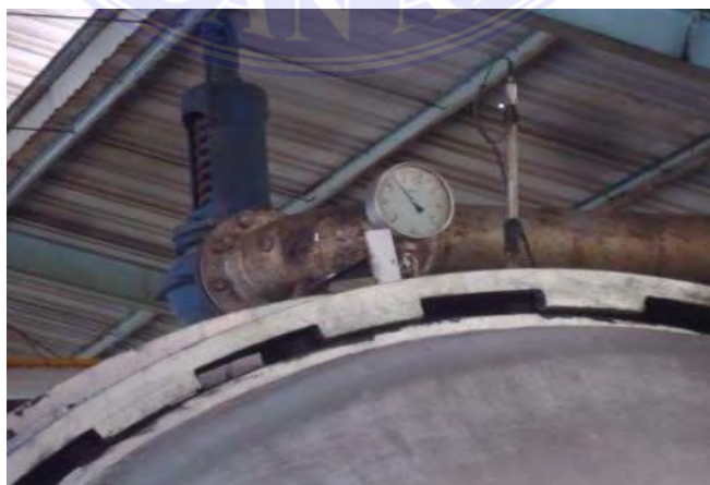
Gambar 3. 6. Katub masuk ( Inlet valve )
