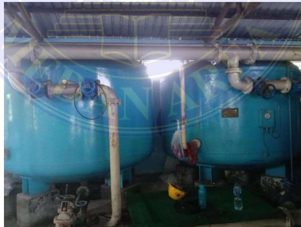
Gambar 3. 49. Sand Filter
