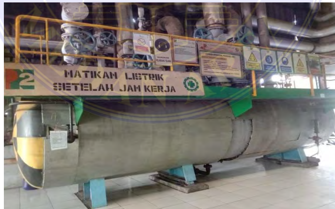
Gambar 3. 55. Back Preassure Vessel
