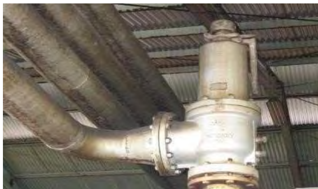
Gambar 3. 4. Katub pengaman ( Safety valve ).
