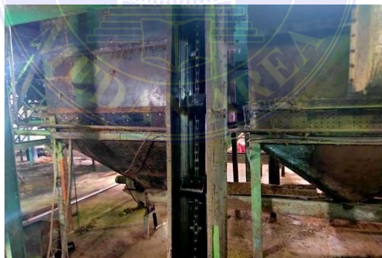
Gambar 3. 36. Wet Nut Elevator
