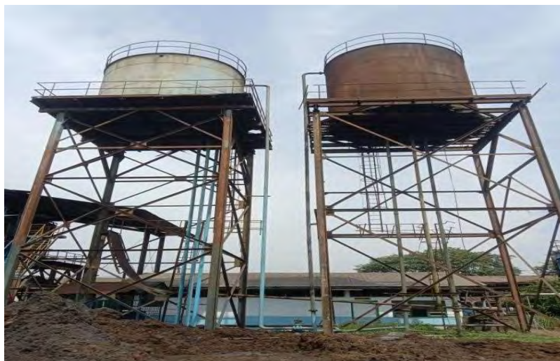
Gambar 3. 50. Water Tower Tank
