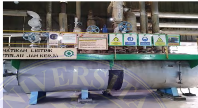
Gambar 3. 52. Back Preassure Vessel
