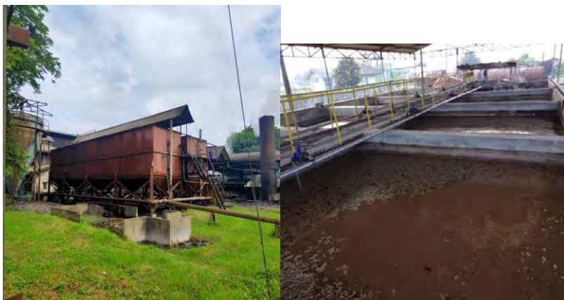
Gambar 3. 55. Bak Recovery Tank
