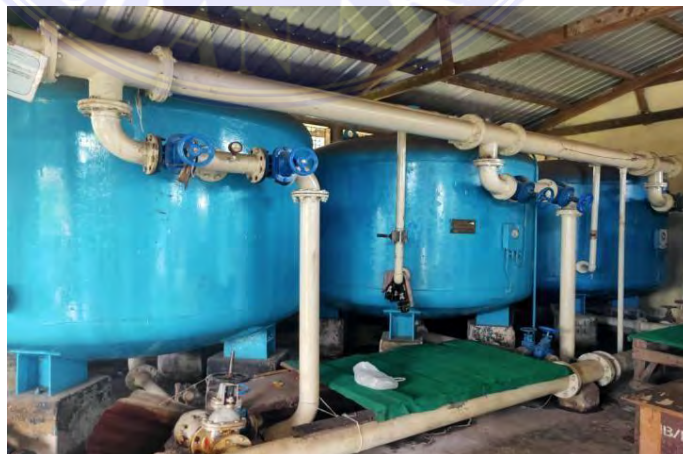
Gambar 3. 46. Sand Filter
