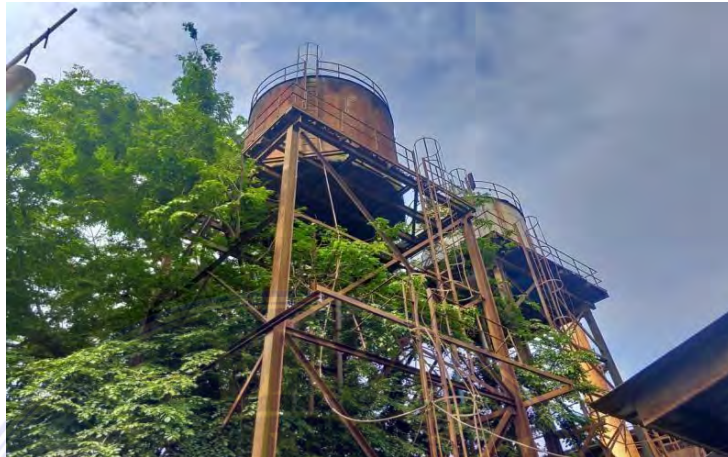
Gambar 3. 47. Water Tower Tank
