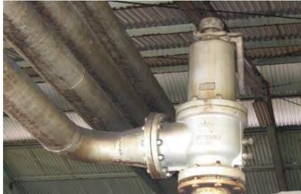
Gambar 3. 6. Katub pengaman ( Safetyvalve )
