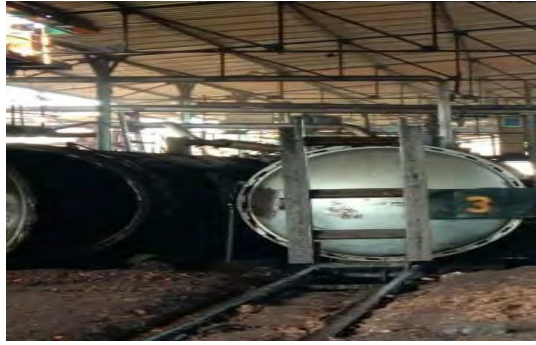
Gambar 3. 13. Jembatan Lori (Cantilever railbridge)
