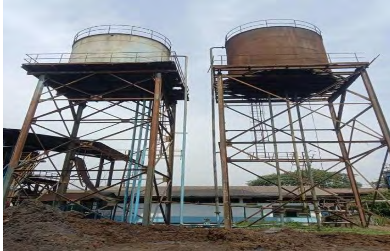
Gambar 3. 50. Water Tower Tank
