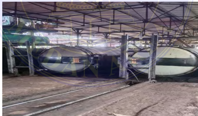
Gambar 3. 11. Jembatan Lori ( Cantilever railbridge )
