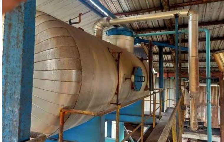
Gambar 3. 52. Daerator Tank
