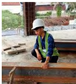
Pengecekan Baja WF
