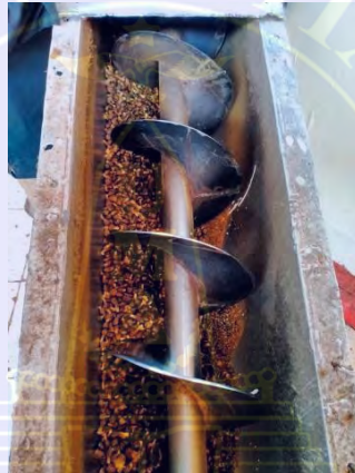
Gambar 3. 33 CAKE BREAKER CONVEYOR (CBC)
