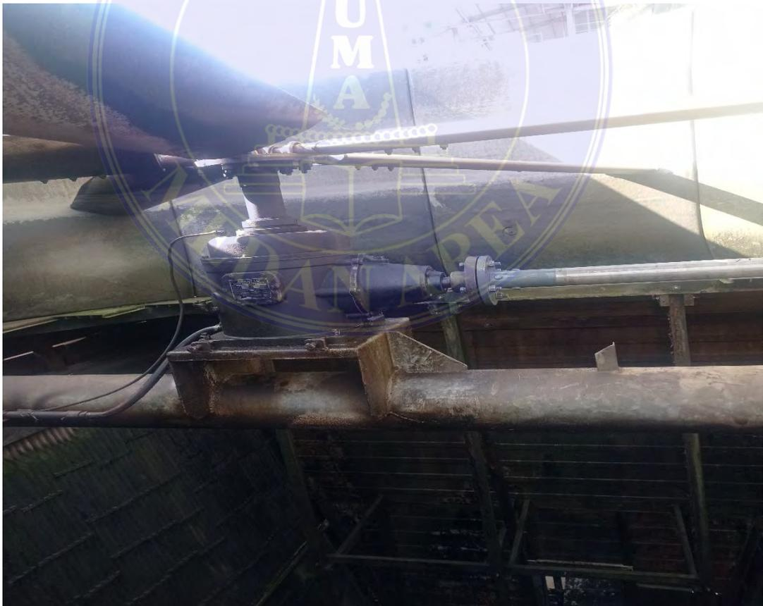
gambar 3. 62 Baling-Baling *cooling tower*
