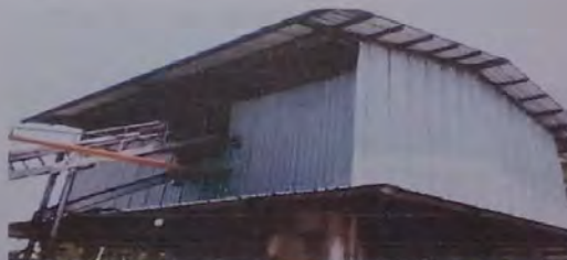
Gambar 3.15. Empty Bunch Conveyor
