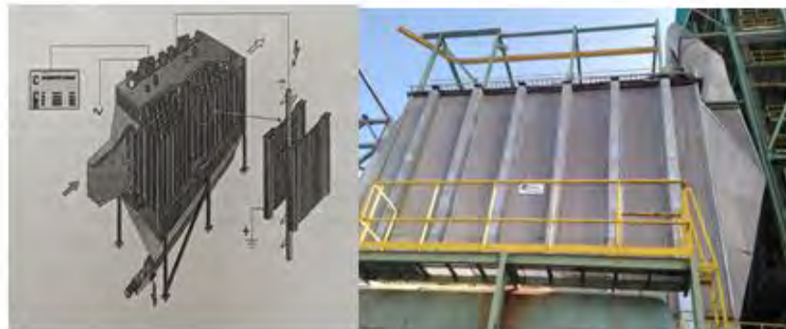
Gambar 2.6 Casing Elektrostatik Precipitator
