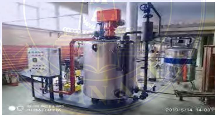
Gambar 3. 57 Boiler Air Panas (*Hot Water Boiler*)
