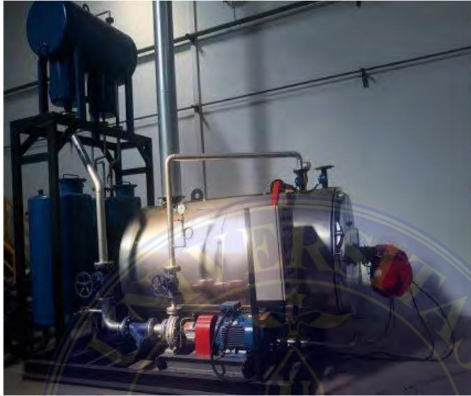
Gambar 3. 60 *Boiler Fluida Termal (Thermal Fluid Boiler)*
