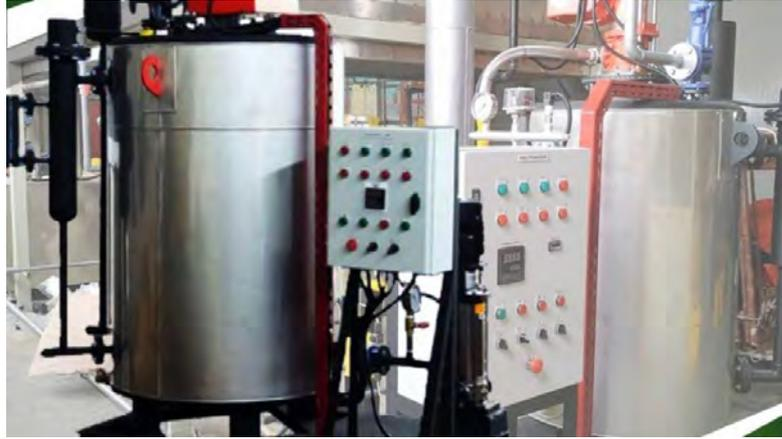
Gambar 3. 58 Boiler Listrik (*Electric Boiler*)
