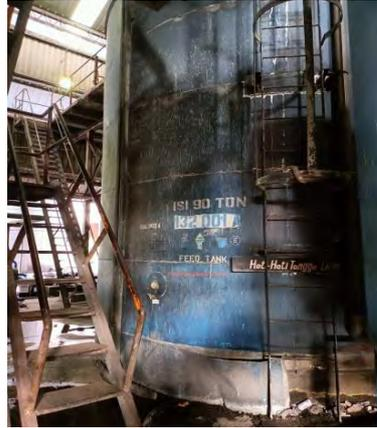
Gambar 3. 48 *Feed Water Tank*
