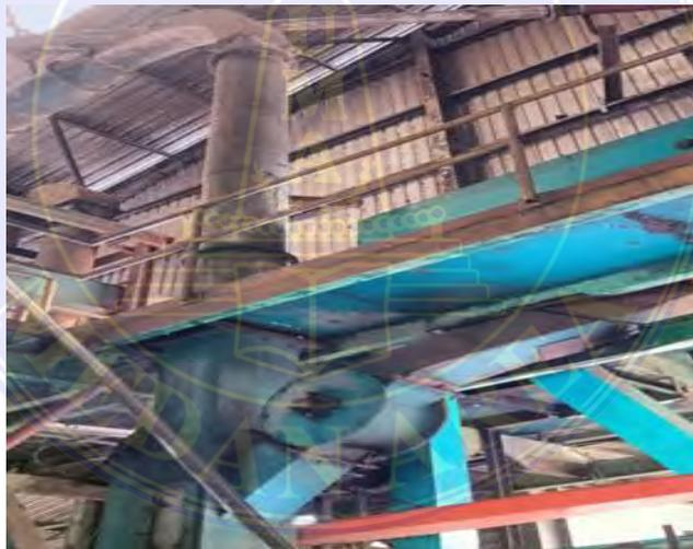
Gambar 3. 39 LTDS (*Light Tenera Dust Separation*)
