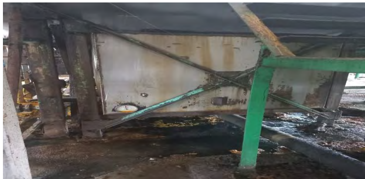
Gambar 3.16. Crude Oil Tank
