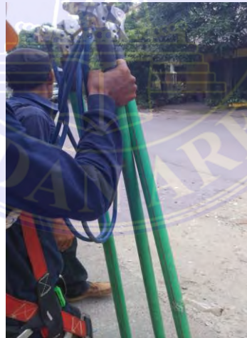
Gambar 3.2 Proses pemasangan grounding.
