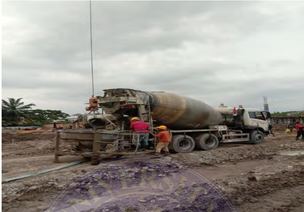
Gambar 4.10. Beton *ready mix* ke *concrete bucket*,
