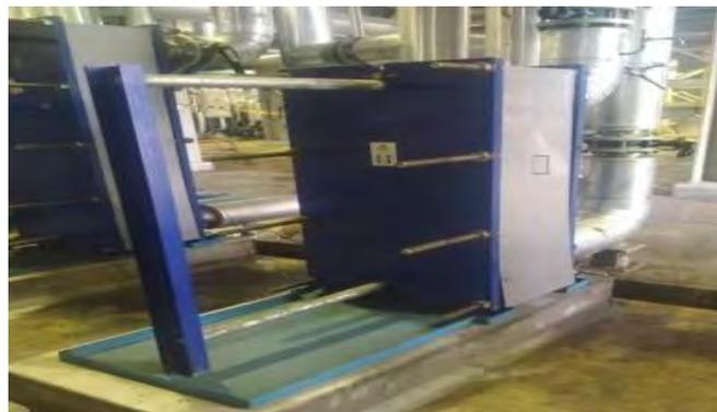
**Gambar 3. 8 *Plate Heat Exchanger***
