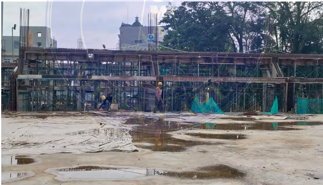
Gambar 8: Bekisting Pelat Lantai Tribun
