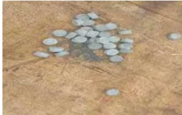
Gambar 3.2.12 Beton Decking
